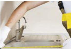
Handmade fabrication templates are created to accurately transfer the measurements and configurations from the job site to the fabrication shop. The most common items used are thin plywood, luan strips and cardboard. Job drawings containing the specific job information and are very important to support the actual template.
